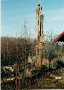
drilling off the waterwell
